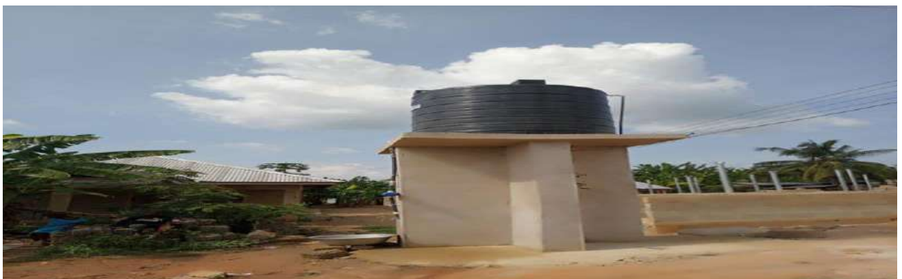
7NO. MECHANIZED BOREHOLE CONSTRUCTED
