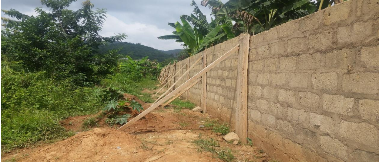
Fence wall constructed CKC SHS, Akaporiso
