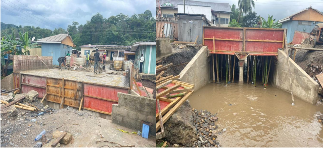
80% work completed on 2m x 2m double box culvert at Kwabrafosso.
